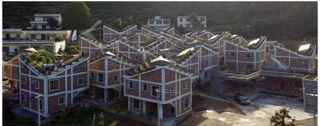
The Jintai Village features an innovative roof design which responds to dense planning requirements by allowing for greater natural light and ventilation. The roof also provides individual household farming.
