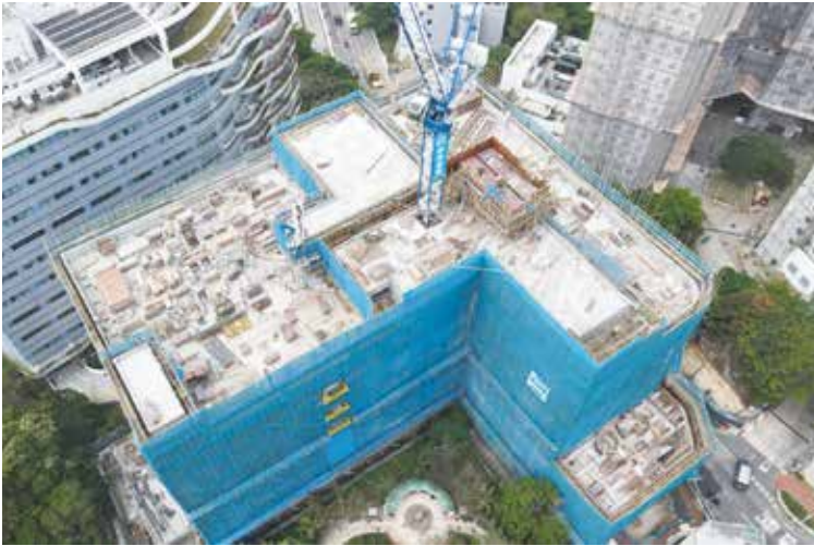
Academic Building at No. 3 Sassoon Road under construction, HKU 港大施工中的沙宣道 3 號教學大樓
