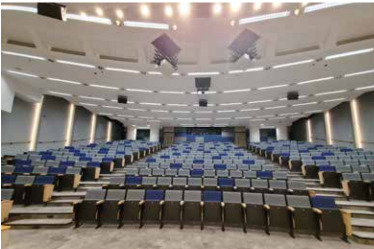
Improvement works of lecture theatres A-H at Academic Concourse 1/F, Zones C, D & E, HKUST 科大學術廊 C、D 及 E 區 1 樓演講廳 A-H 改善工程
