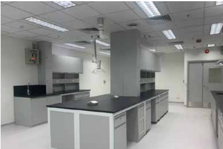
Conversion of English Language Centre into wet laboratories on 2/F of Yeung Kin Man Academic Building, CityU 城大英語中心改建為實驗室工程 (楊建文學術樓二樓)
