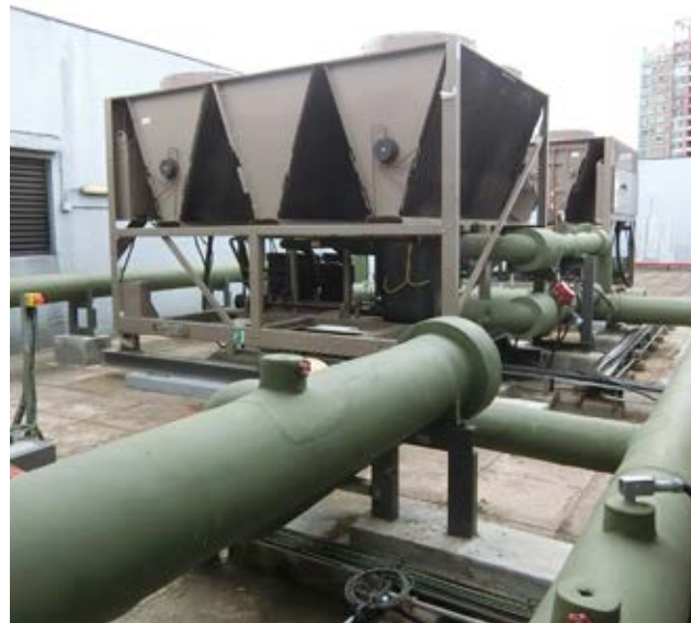
Replacement works of chiller units, chilled water circulation system and building management system for the mechanical ventilation and air conditioning installation, LU 嶺大製冷裝置、冷凍水循環系統及樓宇管理系統更換工程
