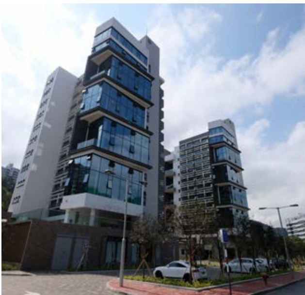
Student hostels on northern campus (blocks A3 and A4), CUHK 中大校園北陲學生宿舍 (A3 及 A4 座)
