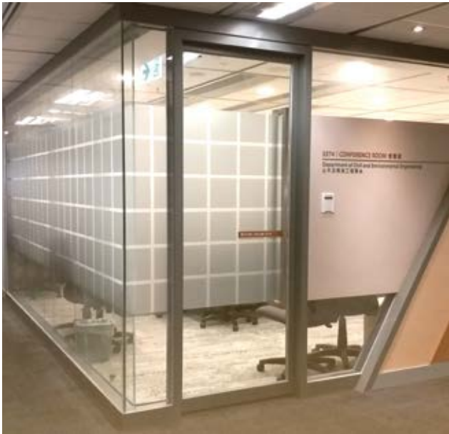
Office remodeling on 2/F and 3/F at Zone E of the Academic Building, HKUST 科大教學大樓 E 區 2 樓及 3 樓辦公室重組工程
