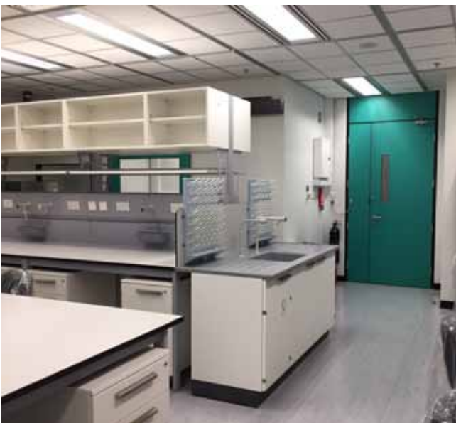
Renovation of laboratory space for research, HKUST 科大實驗室空間改善工程
