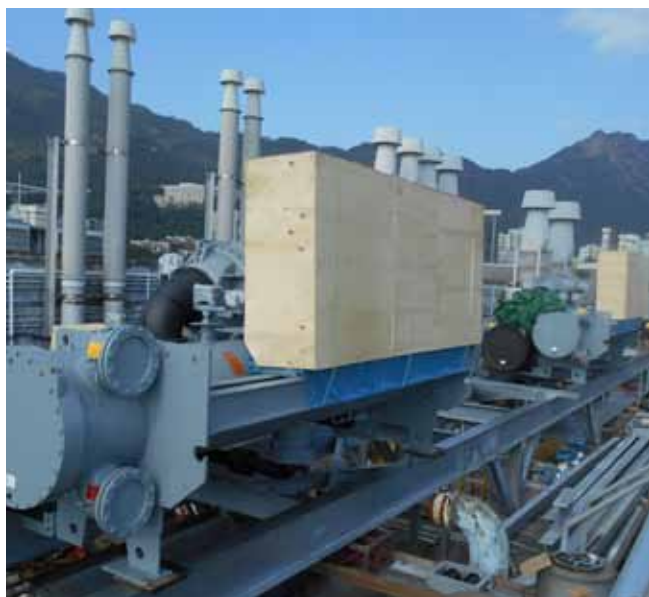
Replacement of air-cooled chillers by water-cooled chillers, CityU 城大以水冷式製冷機替代氣冷式製冷機工程
