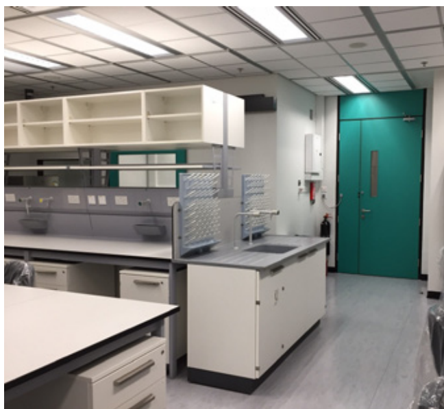
Renovation of laboratory space for research, HKUST 科大實驗室空間改善工程
