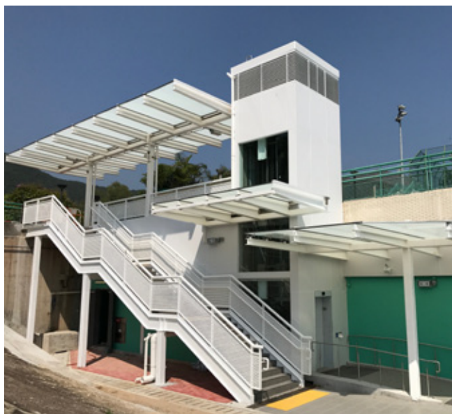
Barrier-free access facilities in Tai Po Campus, EdUHK 教大大埔校園無障礙通道設施
