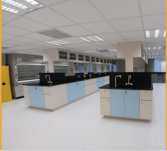
Renovation and improvement works to laboratories at Science Tower, HKBU 浸大科學大樓實驗室翻新及改善工程
