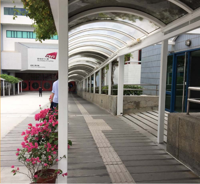
Construction of covered staircase and walkways on campus, CityU 城大有蓋梯級及行人通道工程
