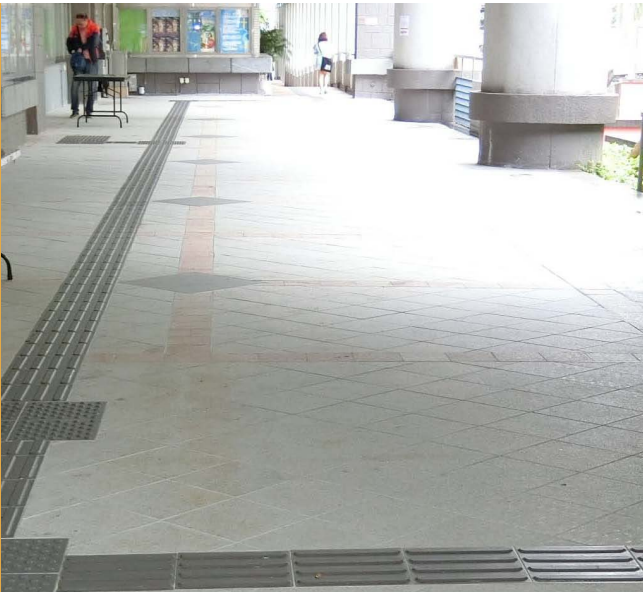
Improvement works to the existing finishes of the pavement within the campus, LU 嶺大校園內行人通道路面改善工程
