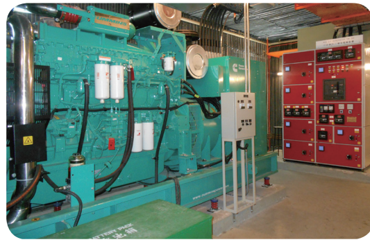
Replacement of aged gensets for Academic 1, CityU 城大學術樓(一)緊急發電機更換工程
