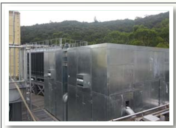
Replacement of air-cooled chillers by water-cooled chillers in block C of HKIEd (AA&I works) 香港教育學院C座製冷機更換工程 (以水冷式替代氣冷式) (改建、加建、維修及改善工程項目)
