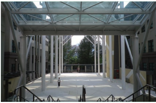
Construction of covered student activities area in LU (AA&I works) 嶺南大學建造有蓋學生活動區 (改建、加建、維修及改善工程項目)
