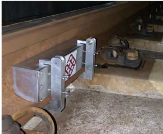
Figure 1: Configurations of Modular Rail Particle Dampers
