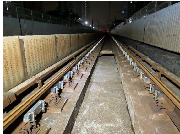
Figure 1: Configurations of Modular Rail Particle Dampers
