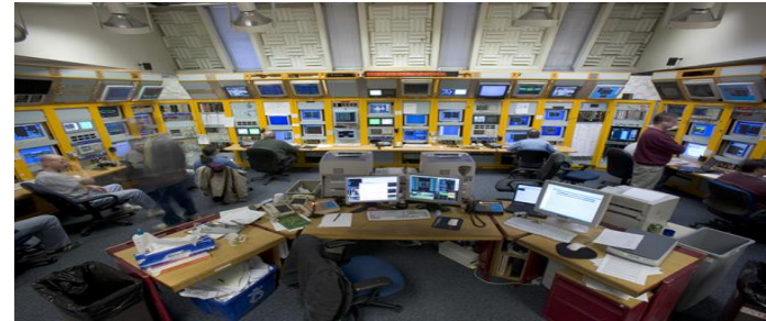
SCADA services http://www.trinitysystems.co.in/
