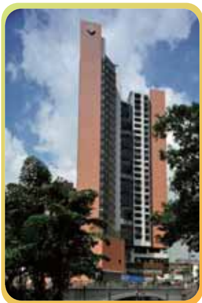
PolyU's newly completed student hostel 理大新落成的学生宿舍
