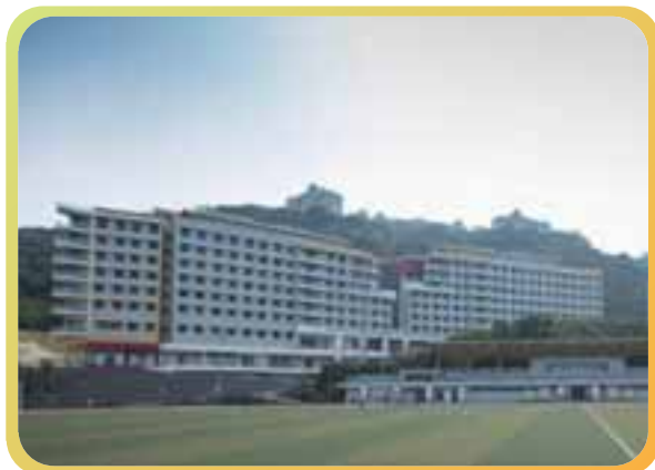
HKUST's newly completed student residences 科大新落成的学生宿舍
