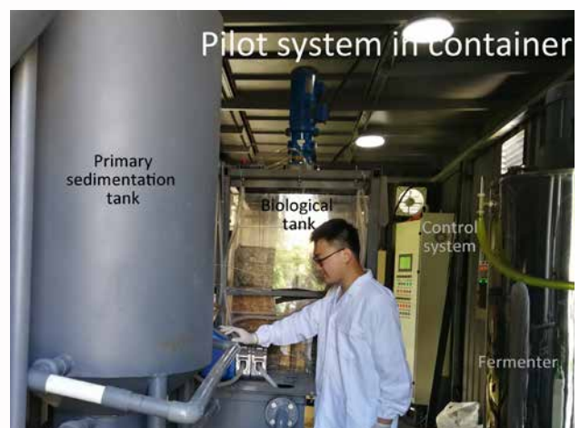
Pilot plant of the advanced wastewater treatment system inside a container tank at Nanshan Wastewater Treatment Plant in Shenzhen, China 測試深圳市南山污水處理廠的集成式污水處理系統
