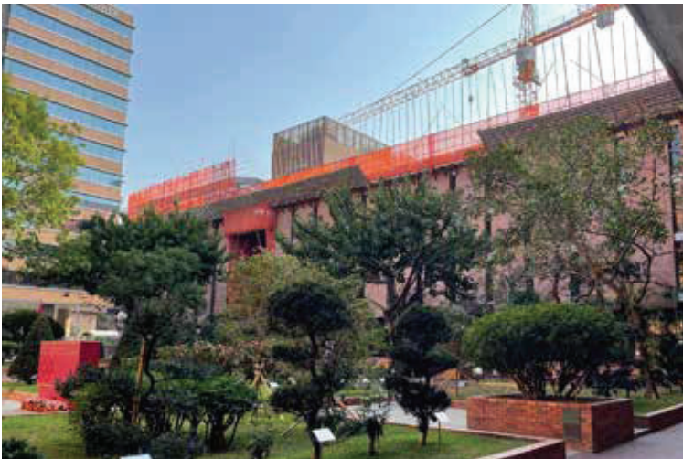
Library Extension and Revitalisation under construction, PolyU 理大施工中的圖書館擴建及翻新工程
