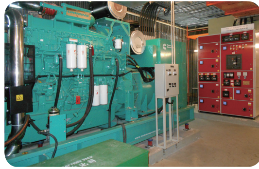
Replacement of aged gensets for Academic 1, CityU 城大學術樓(一)緊急發電機更換工程
