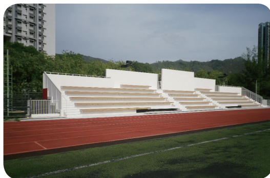
Extension of spectator stand at outdoor sports ground, LU 嶺大戶外運動場觀眾看台的延伸工程
