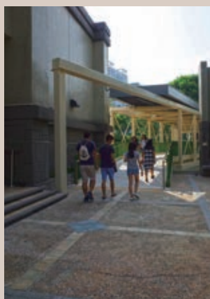
Construction of Footbridge linking the Patrick Lee Wan Keung Academic Building and Indoor Sports Complex to the existing Public Footbridge, LU 嶺南大學建設行人天橋連接李運強教學樓及現有公眾行人天橋工程
