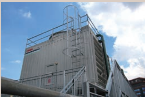
Replacement of existing chiller plant in Phase 5 Building, PolyU 香港理工大學更換五期製冷機組工程
