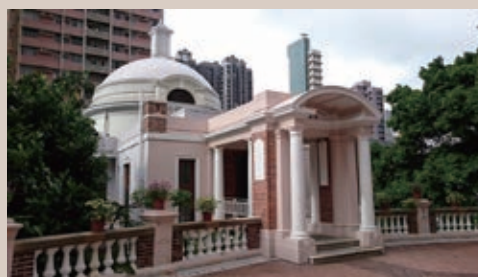
Reorganisation of space at Hung Hing Ying Building, HKU 香港大學孔慶燐樓重整工程
