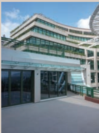
Weather protection cover on G/F at Areas Adjacent to the Central Plaza, HKIEd 香港教育學院中央廣場兩側及通道有蓋空間加建工程
